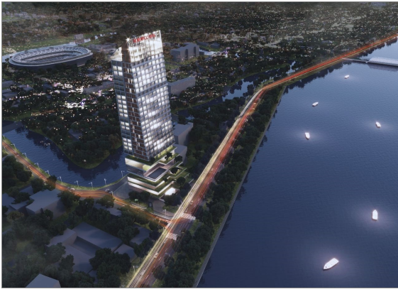
The new Mövenpick Hotel Quảng Bình will overlook the Song Nhat Le River. For high res image please click here .
